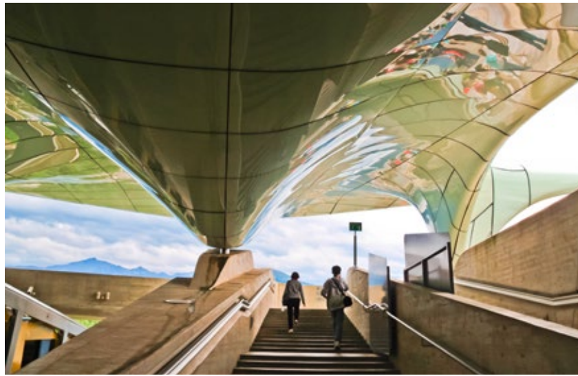
A FUTURISTIC ride up to the high plateau. Exit of the Hungerburgbahn, designed by star architect Zaha Hadid.
