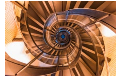
AFTER THE OTHER 133 steps lead visitors to the top of the City Tower.
